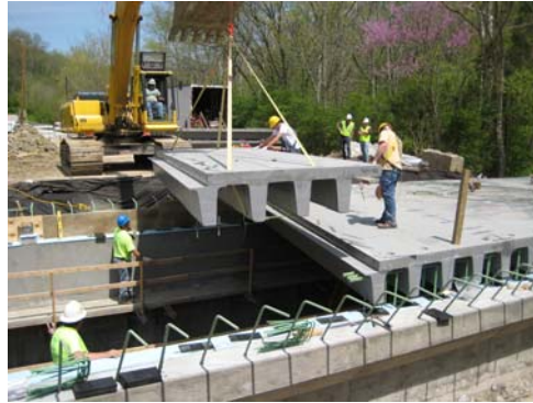
CA FRP panels lowered into place.
