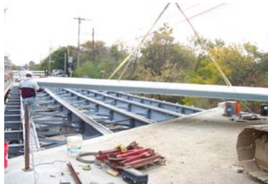
Seventeen composite deck panels were placed in one day.
