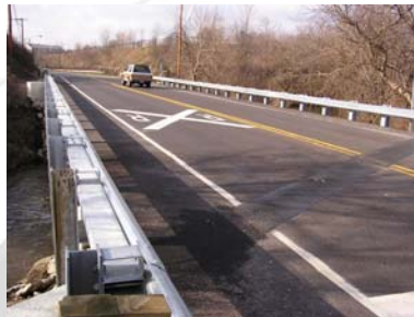
Inspected one month after installation, bridge deck performance has been flawless.
