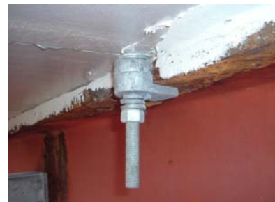
Mechanical fastener connects FRP deck to steel beams.
