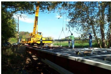
35-ton hydraulic crane helps set panels in place.
